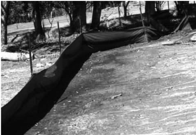
Nutrient filter to prevent contamination of watercourses or storages
